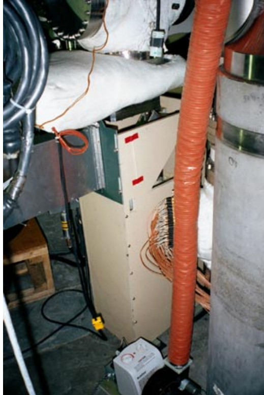
Figure 2-21: The PCI mirror stand underneath the C-Mod tokamak.
