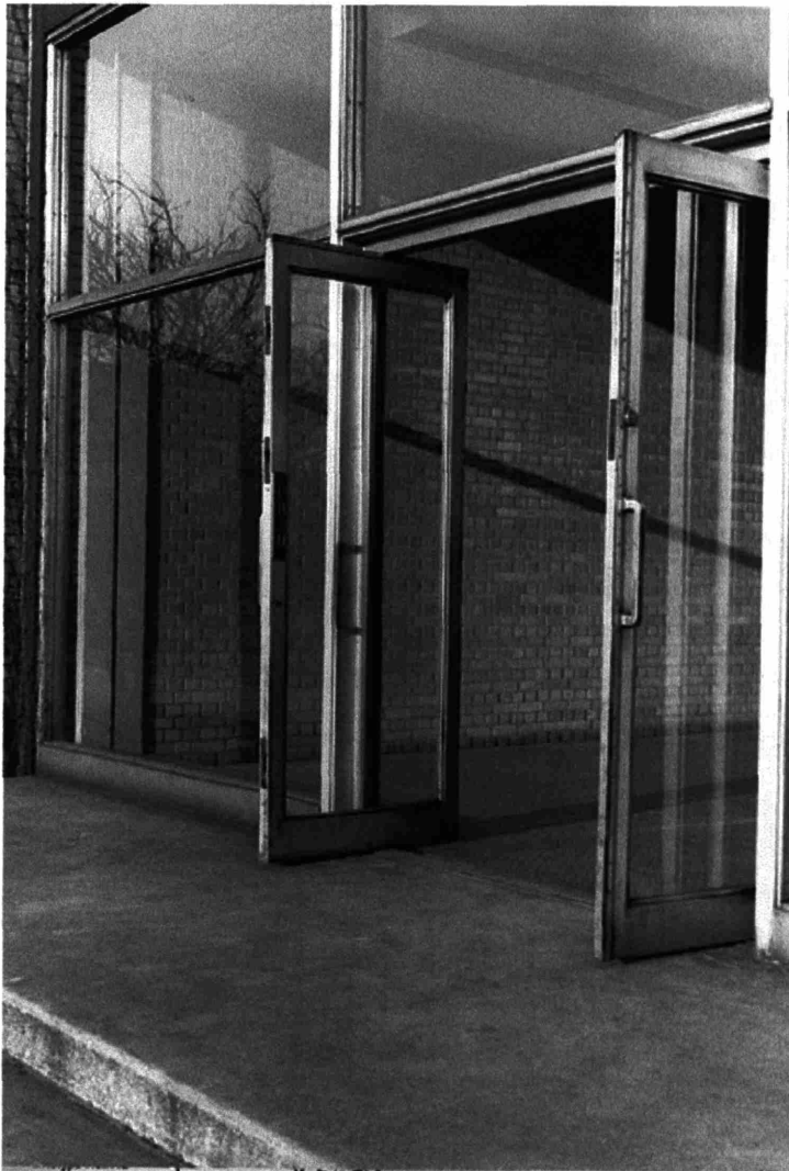
Fig. 3.25: IIT Chemistry Building, 1965.
