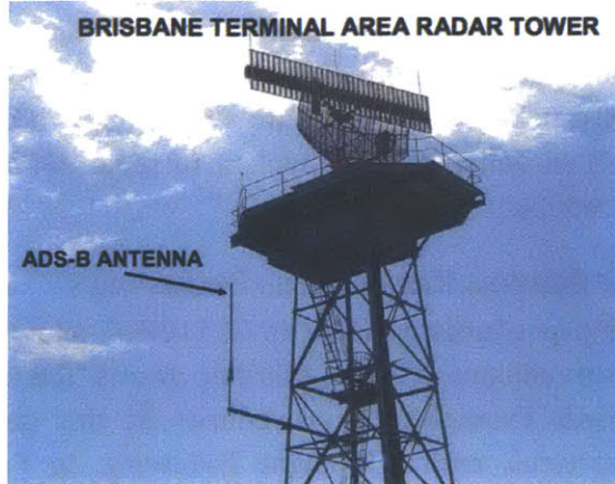
Figure A-4: Temporary Installation of an ADS-B Antenna on a Terminal Area Radar Tower in Brisbane, Australia (credit: Greg Dunstone)
