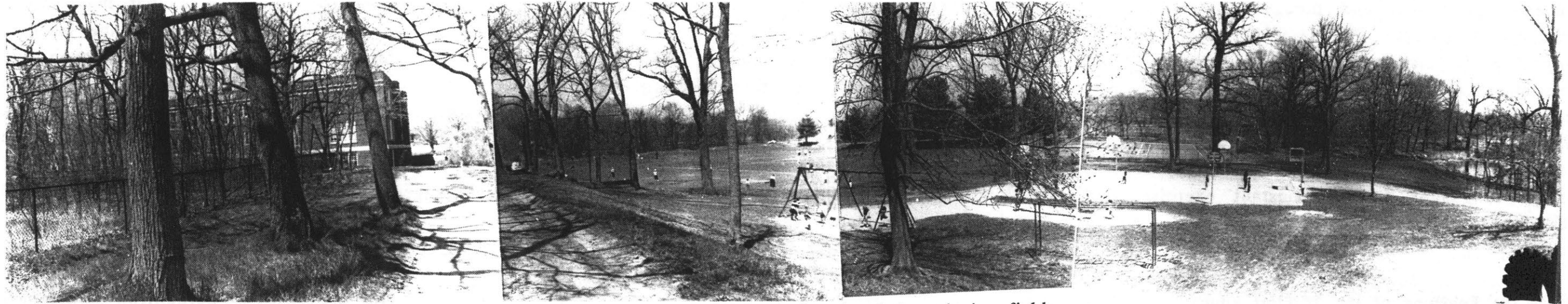
Above is existing school building to be demolished
