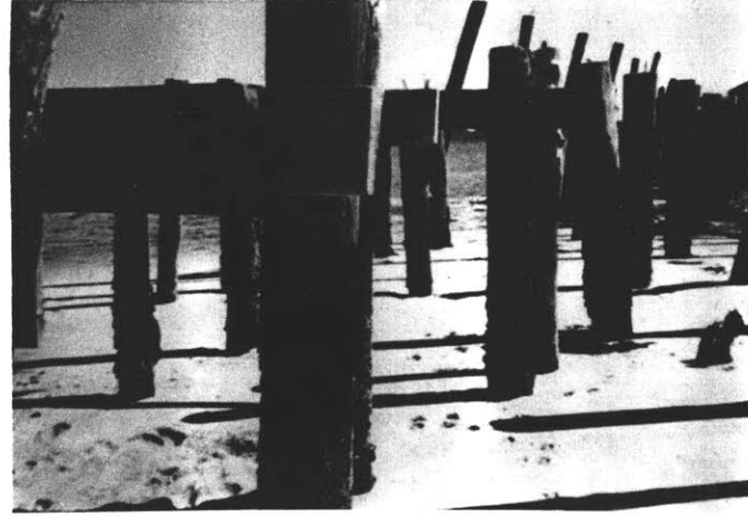
old pier--bay side
