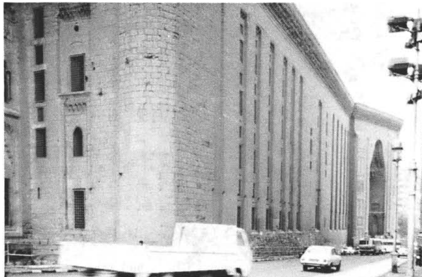
Figure P2.5b: Frame around windows: Madrasa-mosque of Sulṭān Ḥasan. Main facade.
