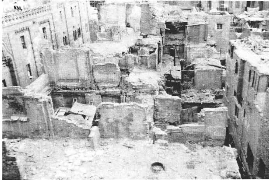
Figure A1.10b: Rab'-wakāla of Qaytbāy (at al-Azhar). View of ruined rab' units.
