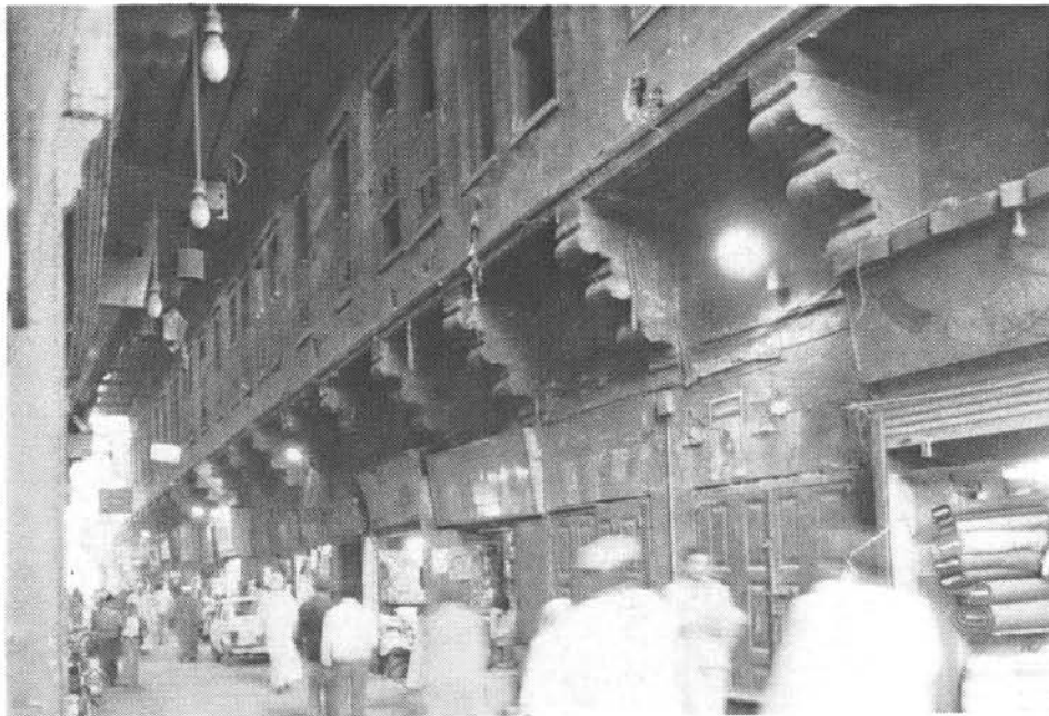
Figure A1.2d: Qasaba of Radwān Bey. View of western rab' , looking south
