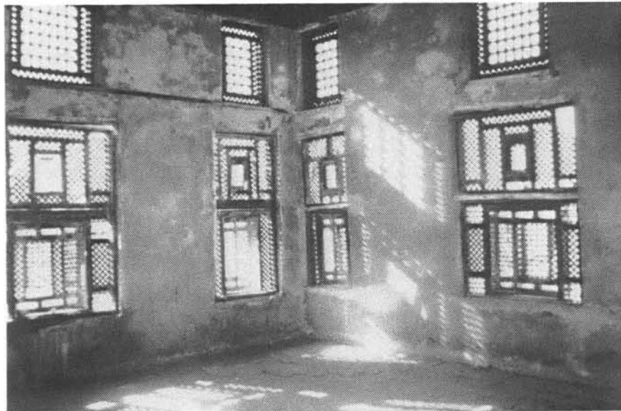
Figure C5.11 Sitting room in Rosetta house.
