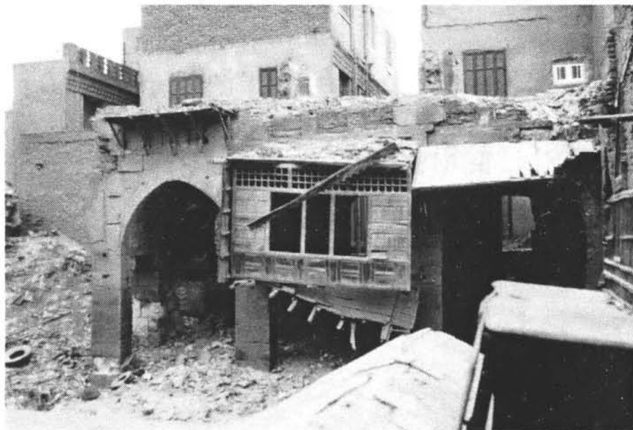
Figure A1.6c: Rab'-wakāla of Qānṣū al-Ghūrī (al-Quṭn). Remains of courtyard.
