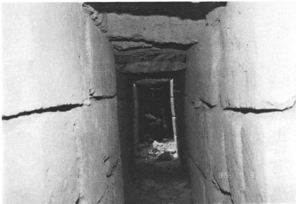
Figure A1.12f: Complex of Ināl. Drainage culvert running underneath rab' block.
