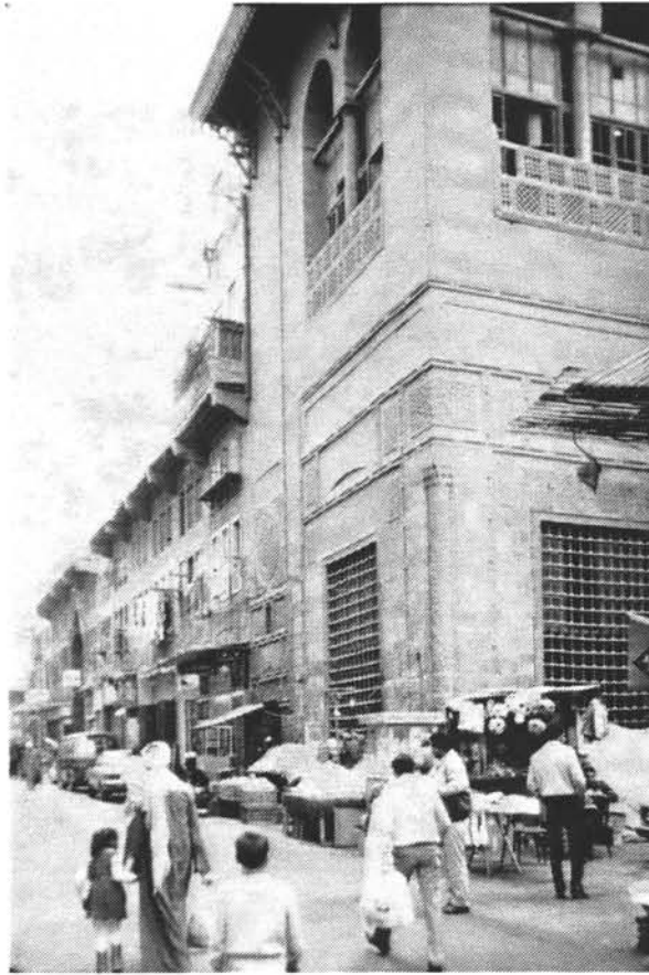
Figure A1.10c: Rab'-wakāla of Qaytbāy (at al-Azhar). Street view looking east.
