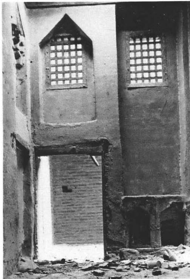
Figure A1.2k: Rab' of Radwān Bey. Skylight in dūr-qā'a .
