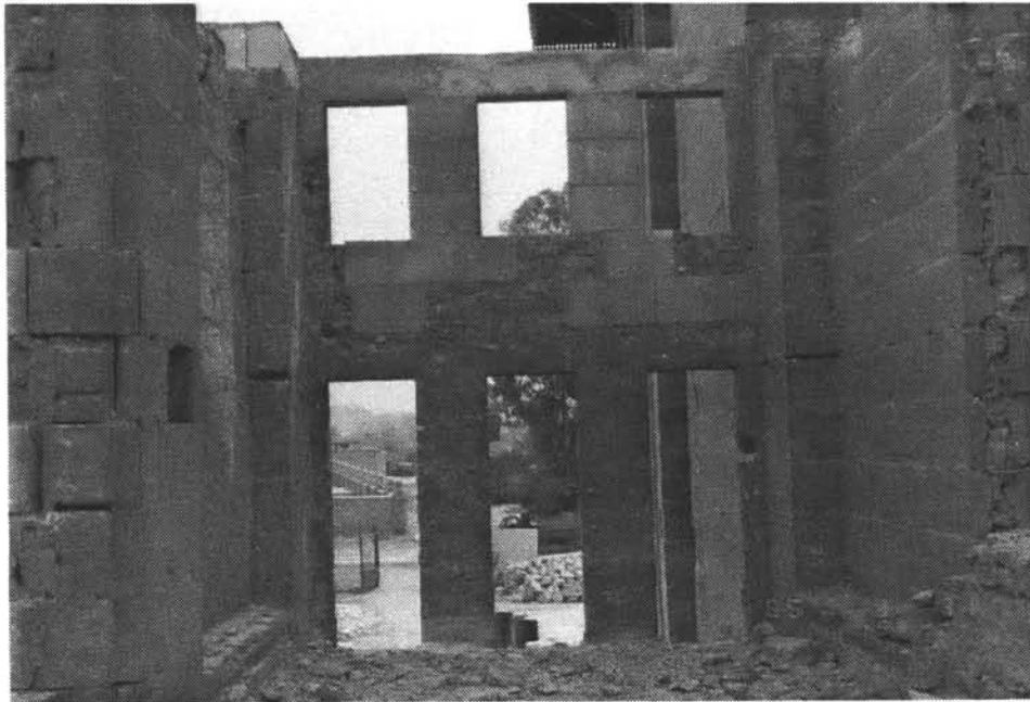
Figure A1.7e: Complex of Qurqumās. Īwān with windows in khanqā .
