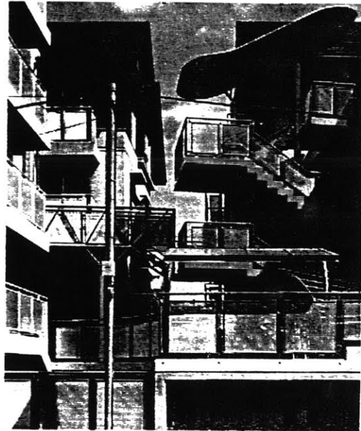
Figure 2 - 32: Ageo, Structure elements are distinguishable by colors and materials
