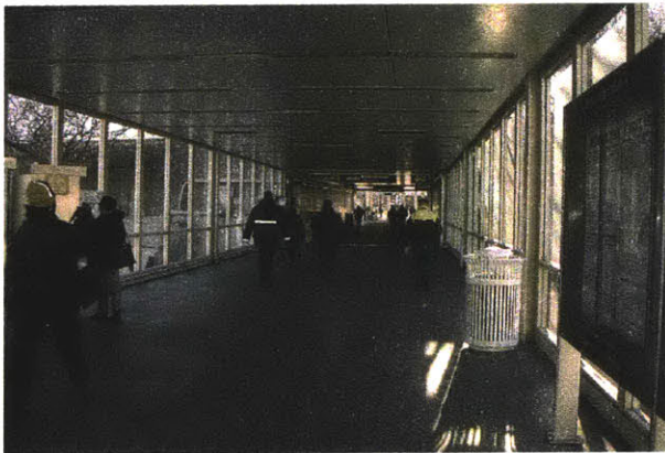
Figure 5-9 From Walkway Under Metra Embankment Toward Station
