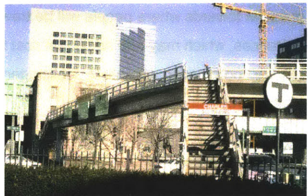
Figure 2-4 Passageway to Entrance of Charles/MGH Station (MBTA)
