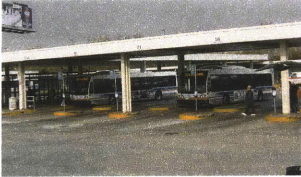
Figure 5-14 Man Using Walkway Across Bus Bays
