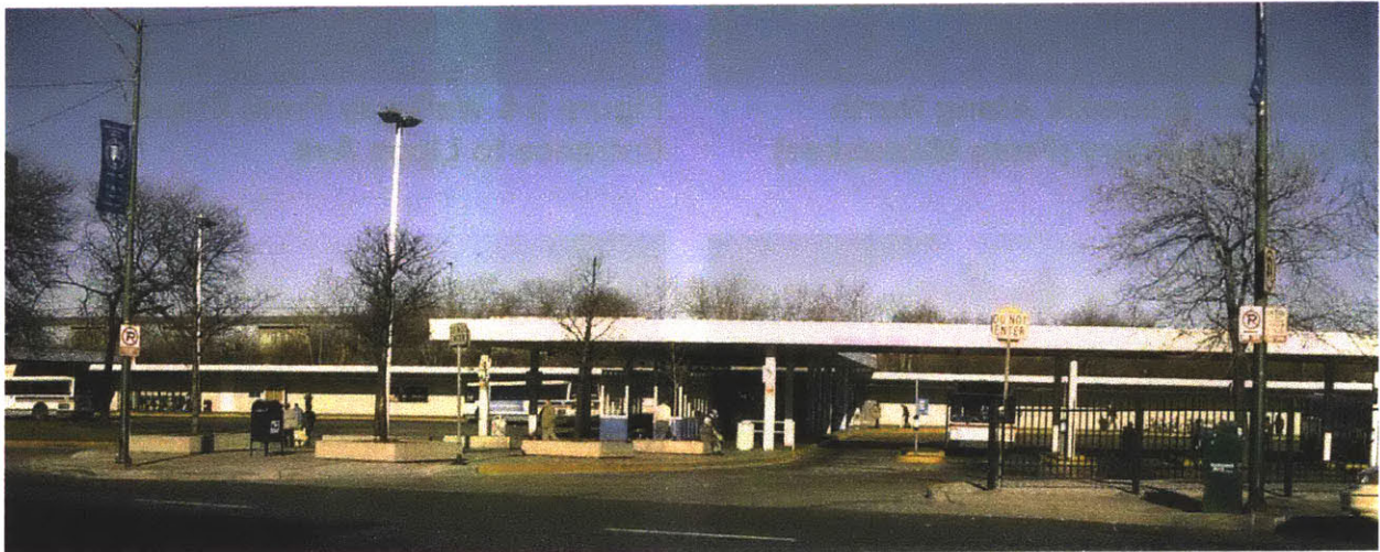
Figure 5-4 From Milwaukee Ave. Toward Station Entrance
