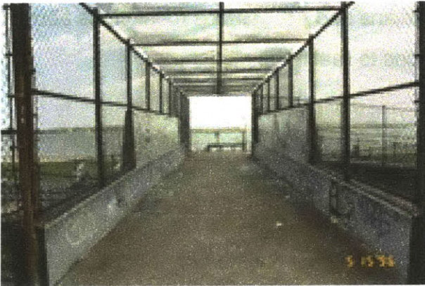
Figure 2-6 Pedestrian Bridge, Before
