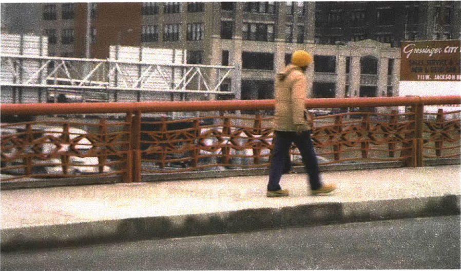
Figure 2-8 Decorative Railing on Bridge Across Expressway
