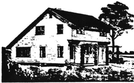
Left: The Colonial "saltbox" house was well-suited to the harsh New England climate. Deciduous vines on the trellis, or "pergola," blocked the summer sun but shed their leaves in winter to permit sunlight to enter the south windows easily.
