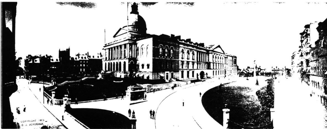
fig. 5.5. The ‘Bulfinch front’ and the completed state house annex. Photograph 1903.
