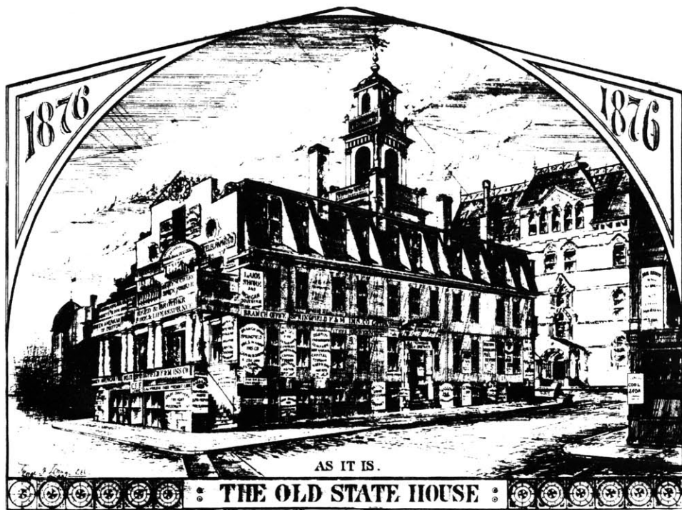
fig. 5.3. 'The Old State House: As It Is.' An 1876 drawing made as part of the preservation effort. Signs cover much of the building's exterior; a mansard roof has been added to increase rentable space. At left, a portico added in 1830 projects into traffic. At right is the Sears Building, a recently-built office block.
