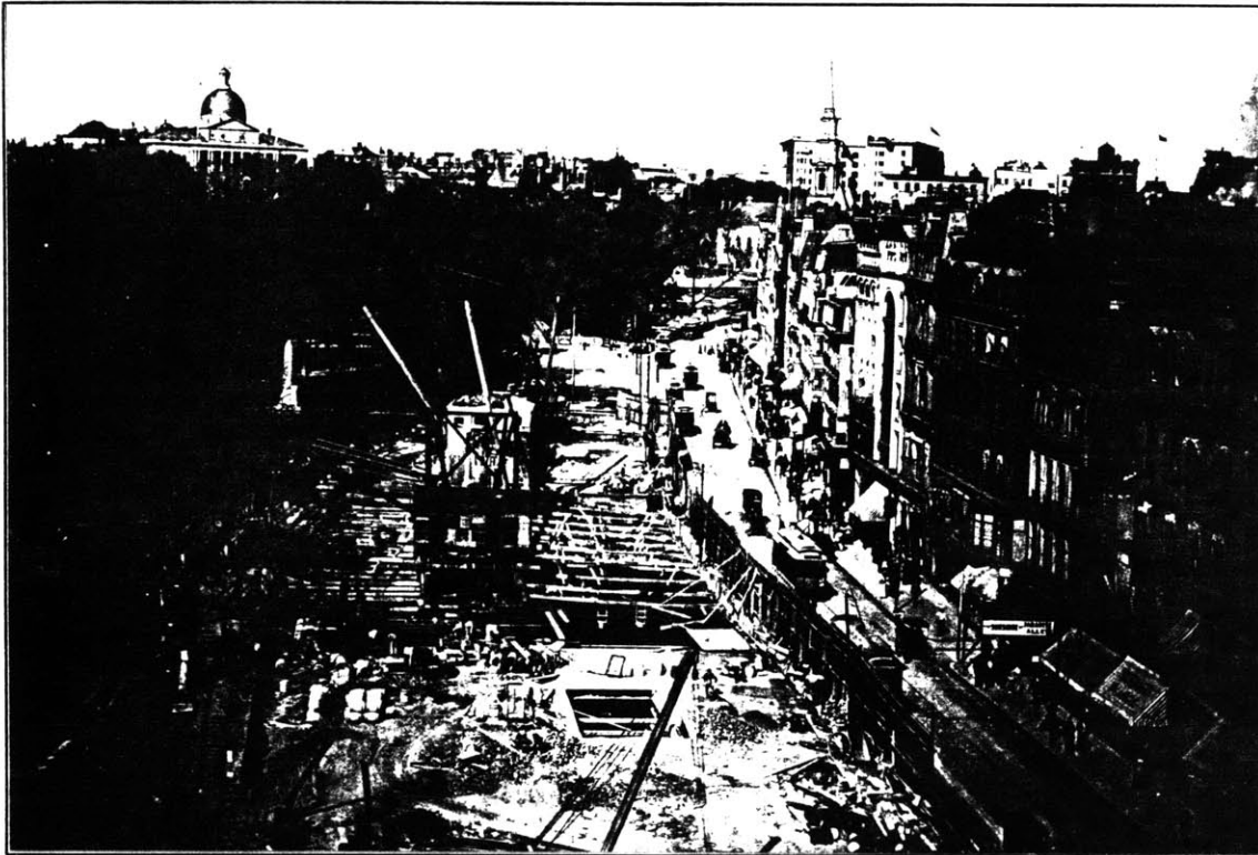
fig. 5.4. Subway excavations under the Tremont Street mall of the Common, 1896. The Bulfinch State House dome and the Park Street Church spire are visible on the skyline.
