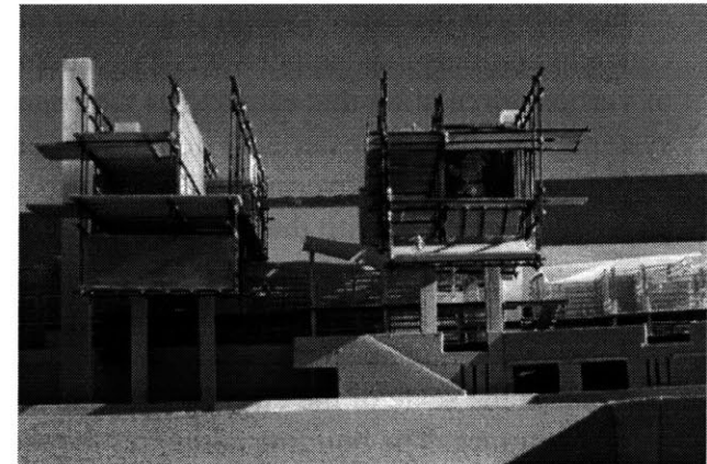
Picture of the Bars without the roof
