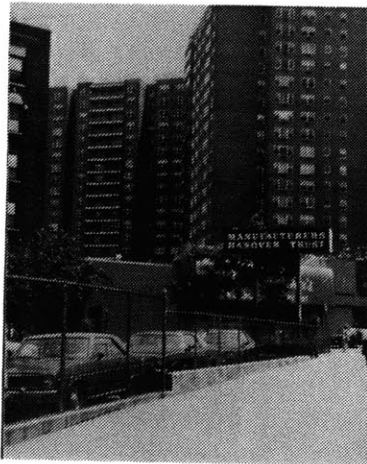
Cluster of apartment towers southeast
