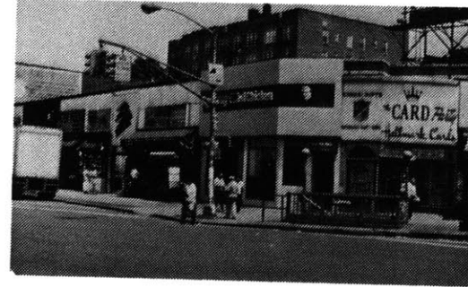
Subway station at the Junction
