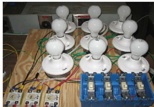
Figure 3: Adjustable test-bed of loads: This arrangement of loads from 75W per phase to 1125W was created for initial testing.
