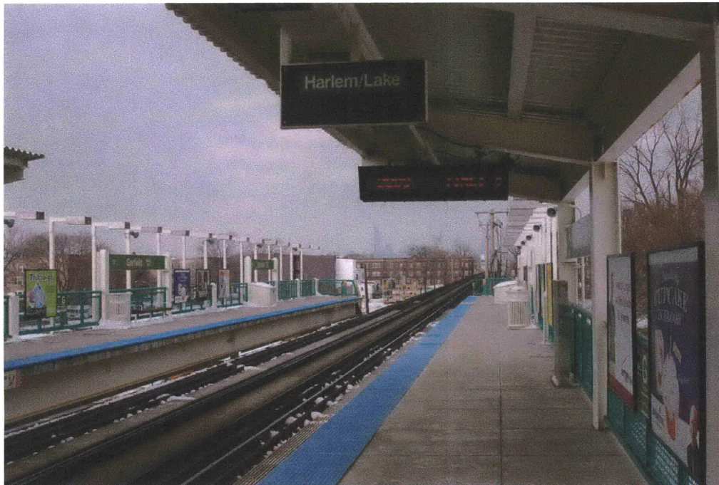
Figure 5.9: Garfield Platform looking towards the Loop. source: Author
