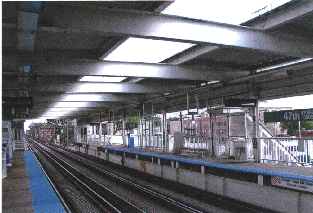
Figure 5.7: 47th Platform , source: Garfield, Graham, http:// www.chicago-l.org/ stations/images/ SouthElevated/ 47th06.jpg
