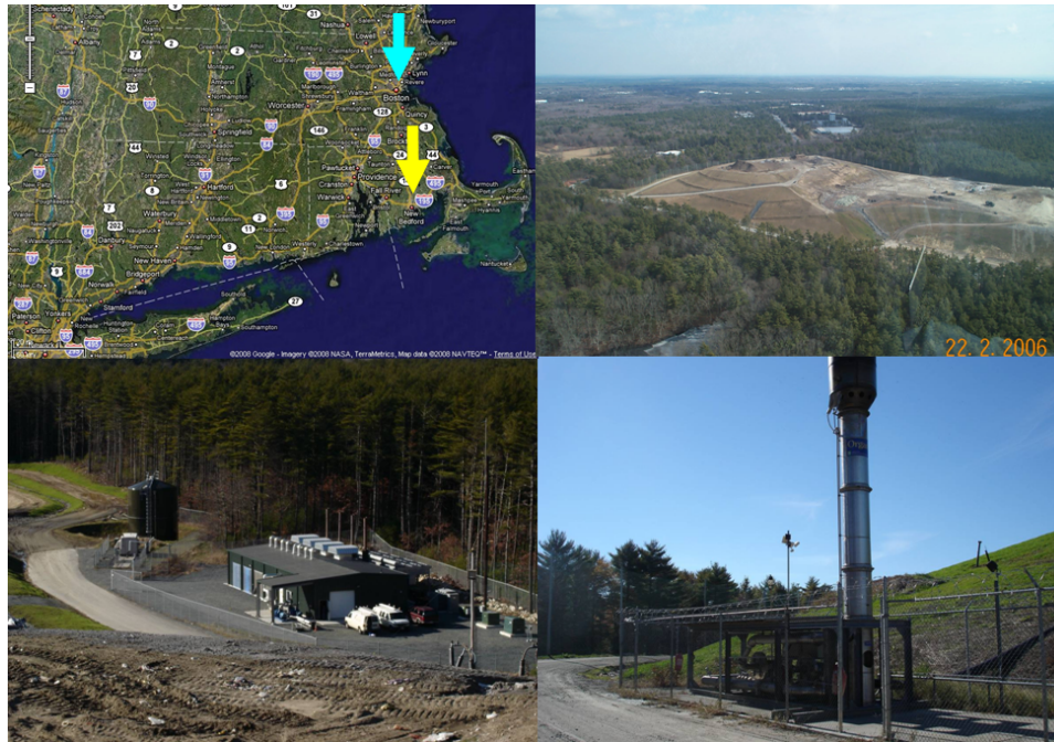
Figure 3-1: Top left: Google Maps image of southern New England. Blue arrow indicates location of Boston. Yellow arrow indicates location of Crapo Hill landfill; Top right: Aerial view of Crapo Hill landfill taken on February 22, 2006 ©Thomas Yeransian; Bottom left: Crapo Hill landfill leachate tank on left and gas to energy plant on right; Bottom right: Crapo Hill landfill flare
