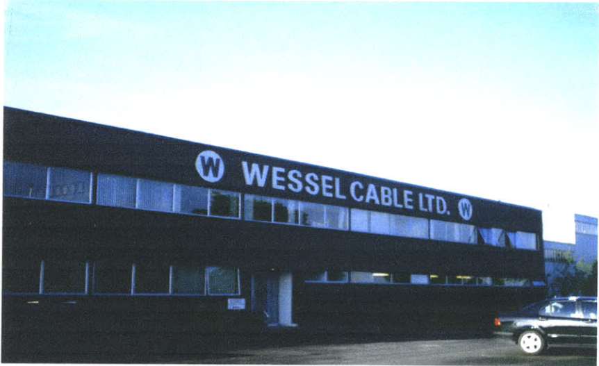
Figure 2-2 ABB Wessel Longford Plant
