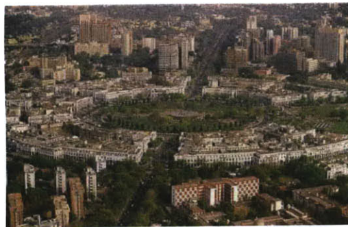
Fig.113 Highrise development, Connaught Place
