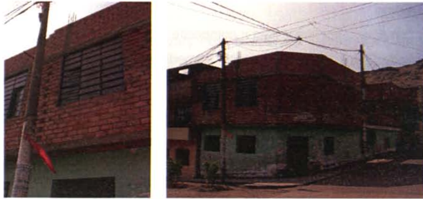
Figure 5.4 Source: Field Work
