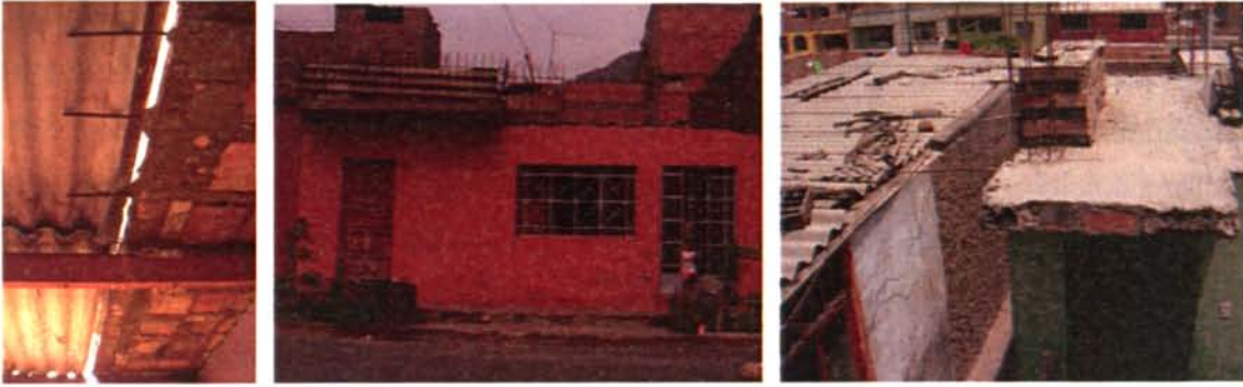
Figure 5.2 – Partial Roof Slabs
