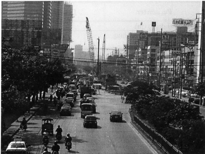
Figure 11.6 Location of the tunnel in Zone 24 (Pracharat Bumphen – Sutthisan)
