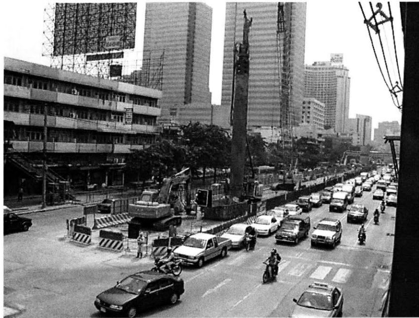
Figure 11.7 Location of the tunnel in Zone 25 (Sutthisan - Ratchada)
