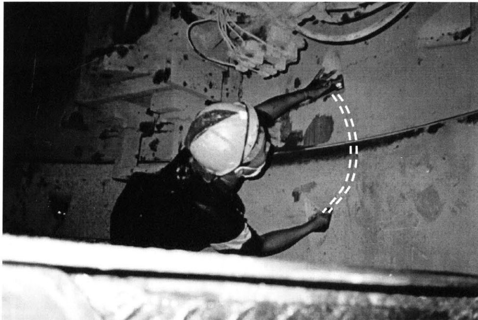
Figure 2.27 Worker securing a curve bolt between segments
