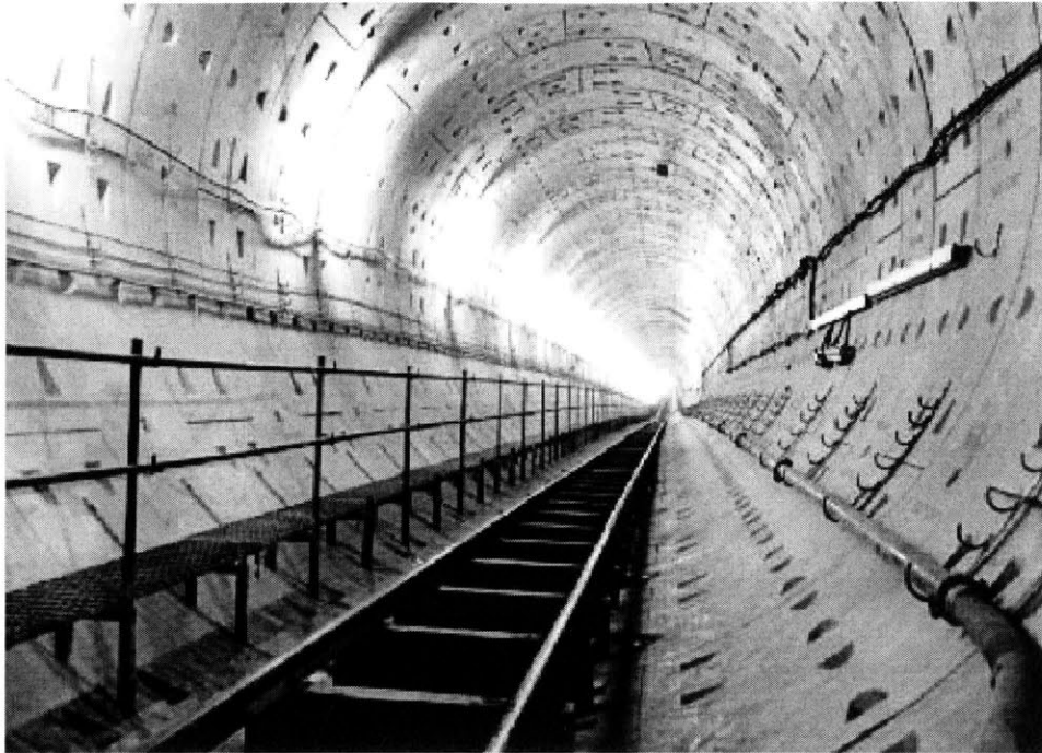
Figure 2.20 The Bangkok MRTA Project, reinforced concrete segmental lining
