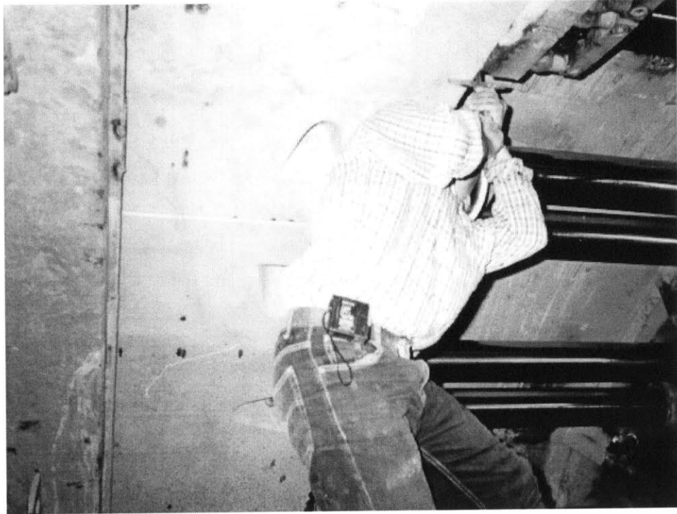
Figure 2.28 Worker checking the position of the installed lining ring
