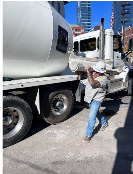
Figure 1 CDP assembling steel chutes before pouring concrete in Boston, MA.
