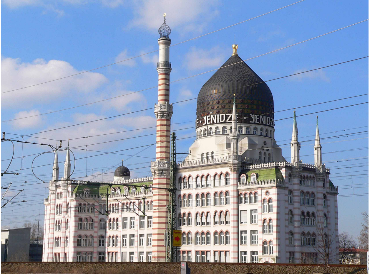
Figure 3.8 The Yenidze Oriental Tobacco and Cigarette Factory after its 1997 reconstruction program. Image via ID Historische Friedrichstadt.
