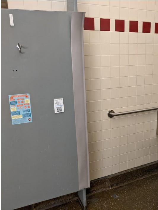
Figure 4.9: Additional privacy strips covering gaps in conventional restroom stalls with toilets fixtures.
