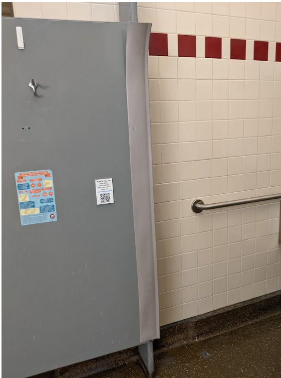
Figure 7.3: Additional privacy strips covering gaps in conventional restroom stalls with toilets fixtures.
