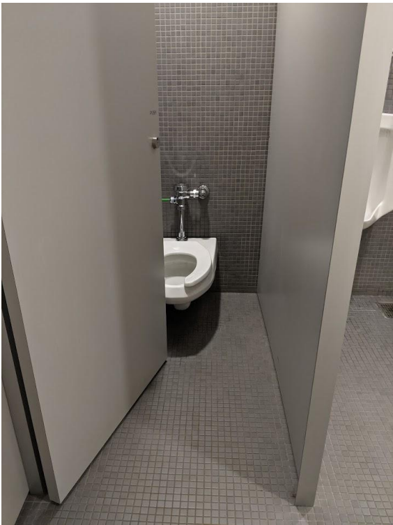
Figure 7.5: Fully enclosed restroom stall with toilet fixture.
