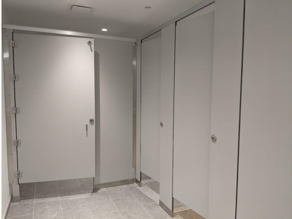
Figure 4.13: Stalls that are taller/go lower than conventional restroom stall. Stall doors also have smaller gaps between the door and the doorjamb than conventional restroom stalls.
