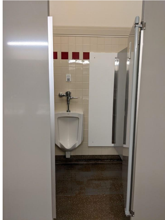
Figure 7.2: Urinal enclosed in its own stall with additional privacy panels (the white and metal strips along the doorjamb).
