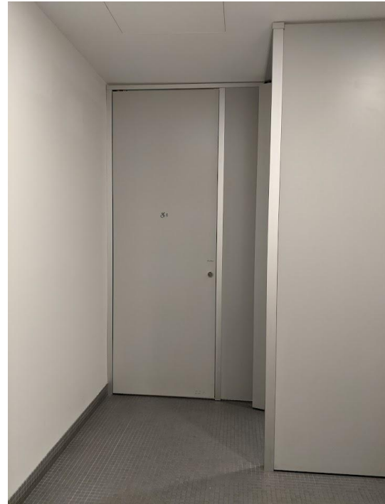
Figure 4.12: Fully enclosed restroom stalls
