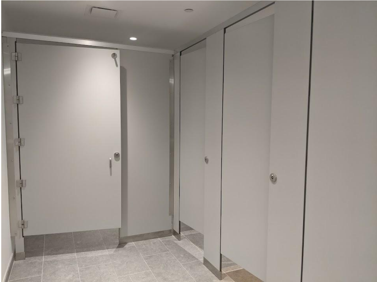
Figure 5.3: High-privacy (but not fully enclosed) stalls implemented in the Hayden Library renovation.
