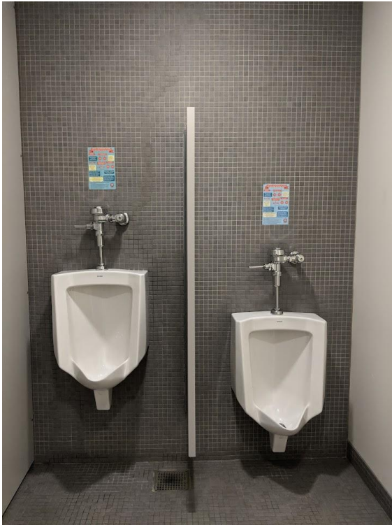
Figure 7.1: Two urinal fixtures separated by a divider; no separate stalls.
