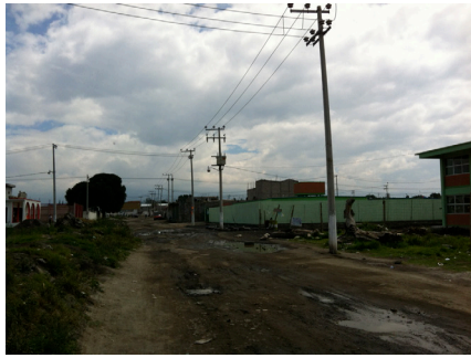
Electricity is usually the first service to arrive.
