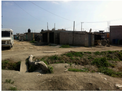
Houses under construction in Chimalhuacán.
