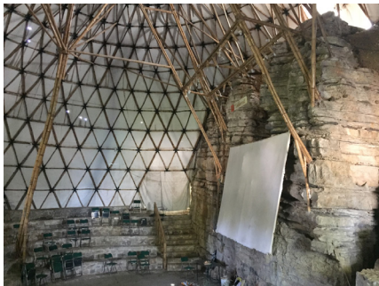
The auditoriom at Tosepan is a geodesic dome with a bamboo structure.
