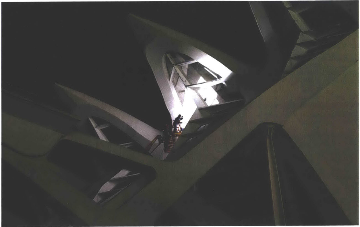
Workers fix leaking windows in the science museum
