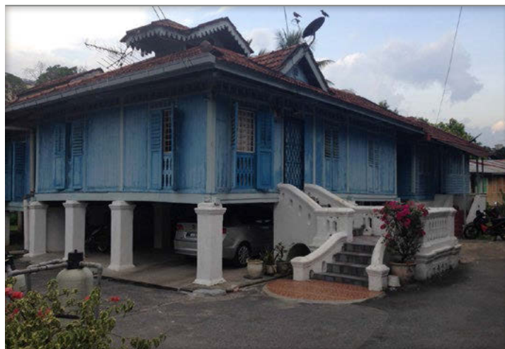
Figure 12. Traditional Malay House in Kampung Bharu. Photo credit: Valeria Vidal Alvarado, 2016
