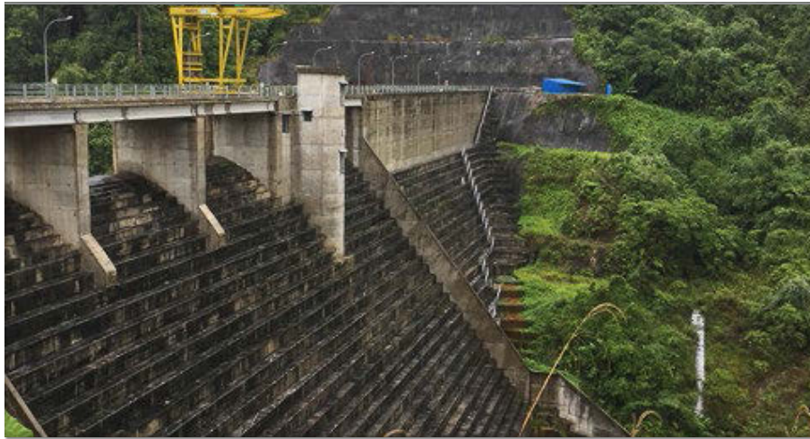
Figure 22. Dam in Kuching. Photo Credit: Lisa Young, 2015
